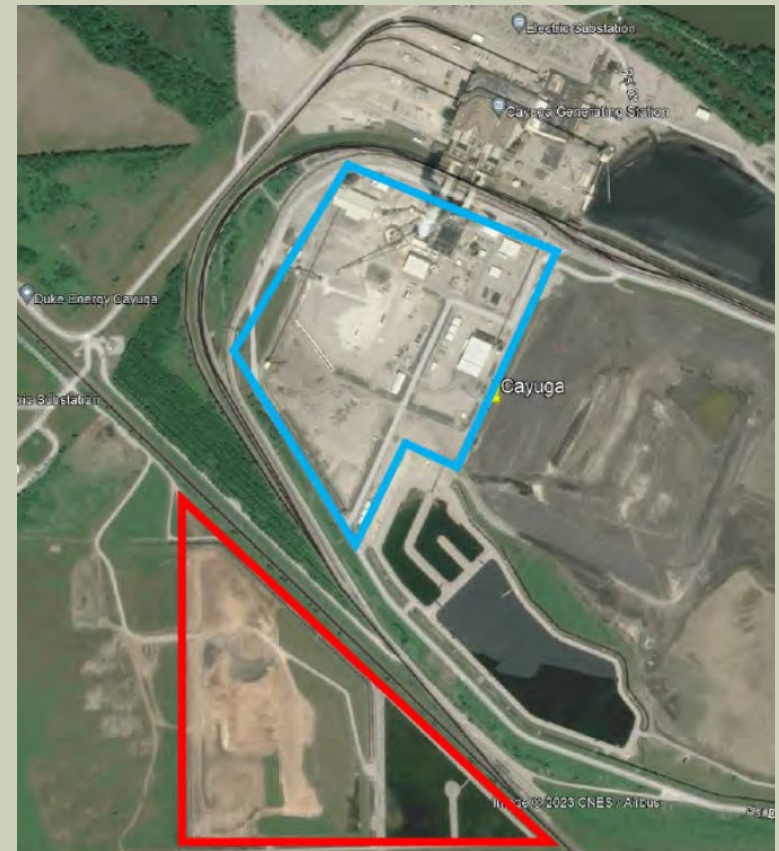
Aerial photo showing two coal ash landfills at the Cayuga power plant. Source: CN 46038, Attachment 19-B (TSH)
